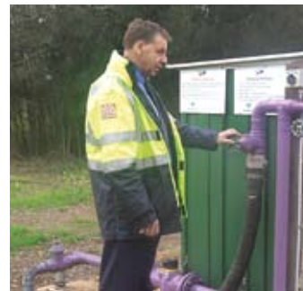
David Allen – CFA Manager, Community Infrastructure for Outer Metro Norwest Region, examines the recycled water standpipe at Surbiton Park.
