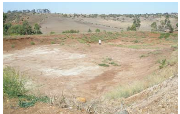
Below: The future site of the 8 ML recycled water storage facility at the Plant.
