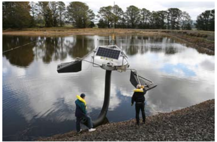
The SolarBee™ is lowered onto Lancefield Basin on 19 August.
