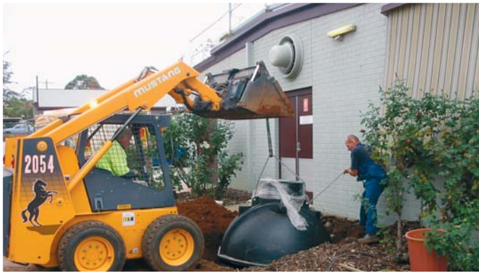
Installation of the underground cooling water tank at Bacchus Marsh Hospital
