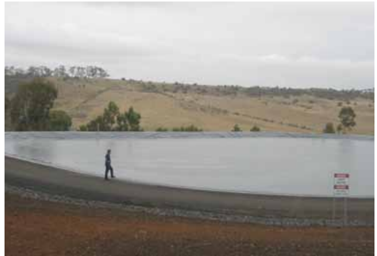
The new storage at Sunbury Recycled Water Plant will secure supply during periods of low inflow and high demand.
