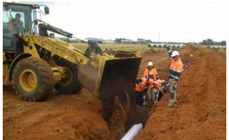
Construction of the new Class A Toolern pipeline commenced on 16 March.
